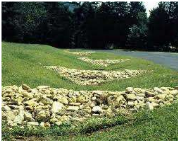
Rock check dams similar to our project
