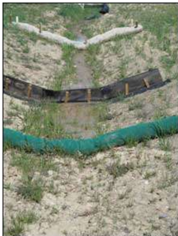
Three samples of straw or fabric check dams
